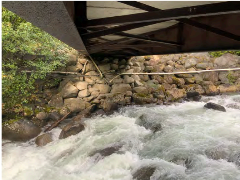
Right Bank Abutment when facing downstream
