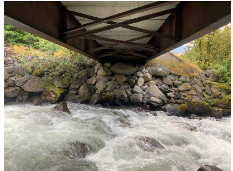
Left Bank Abutment when facing downstream
