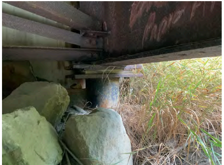
Bearing, left bank
