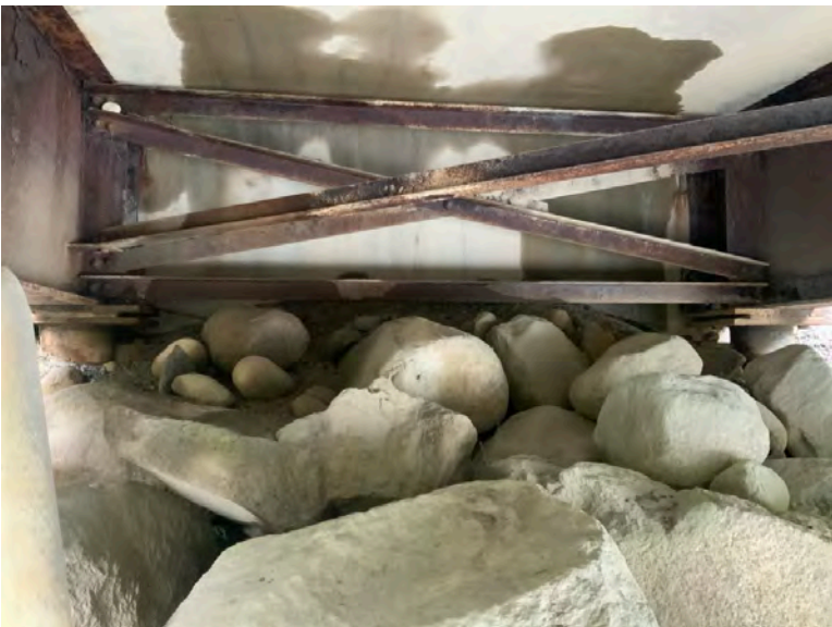
Right Bank Abutment when facing downstream
